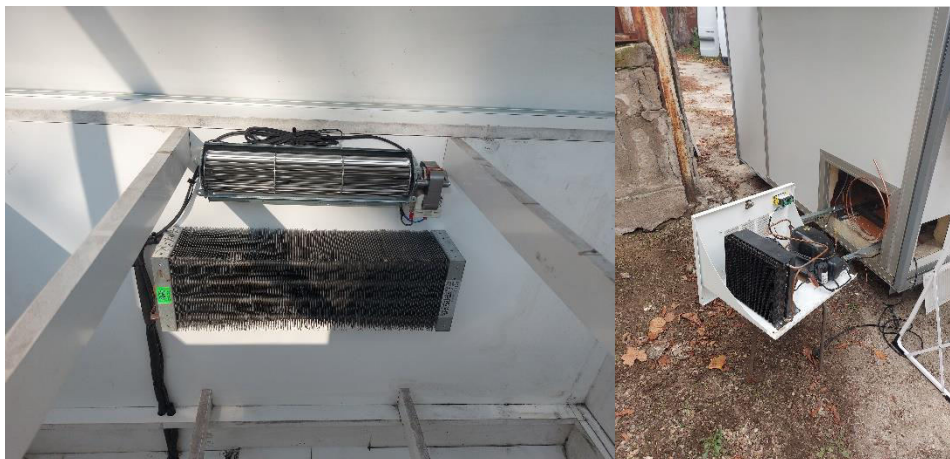
Fig. 9. Refrigeration installation subsystem
