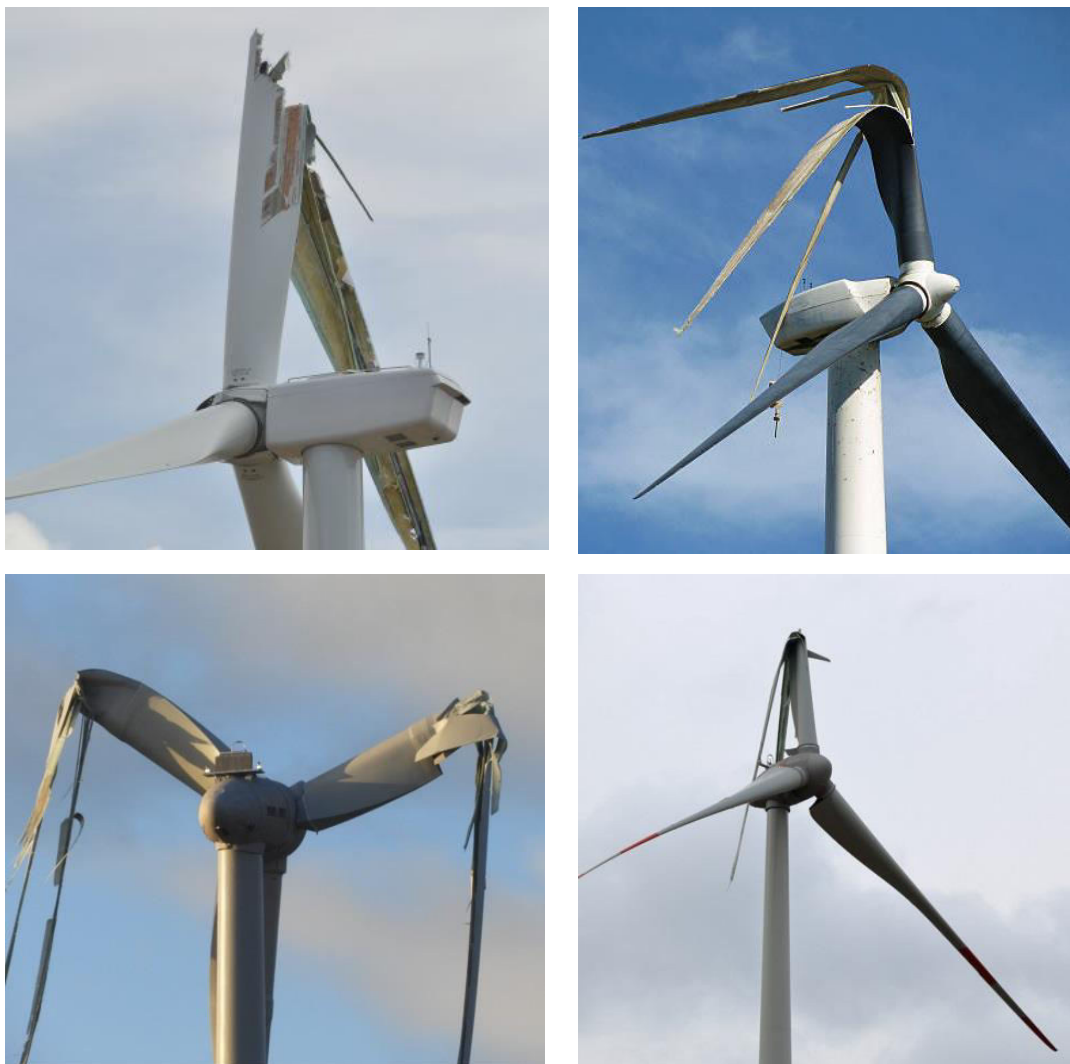
Fig. 2. Location and appearance of damage on operating wind turbine blades
