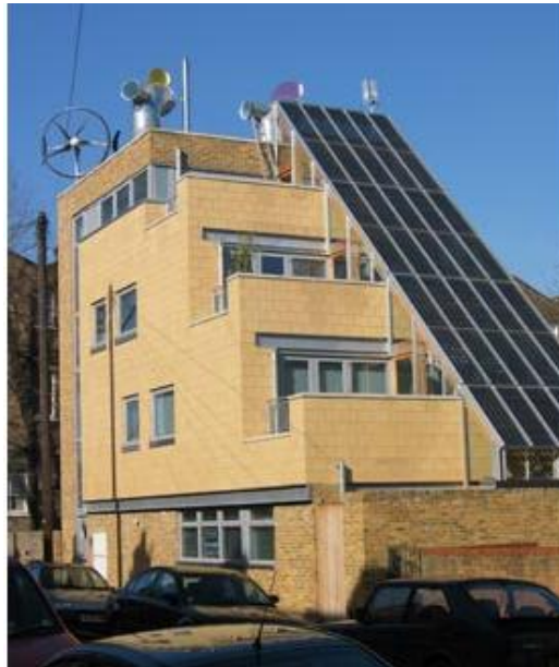
Fig. 4. The influence of the roof in the placement of a wind turbine [5]
