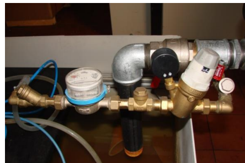
Fig. 7. The connecting pipe of the injector device
