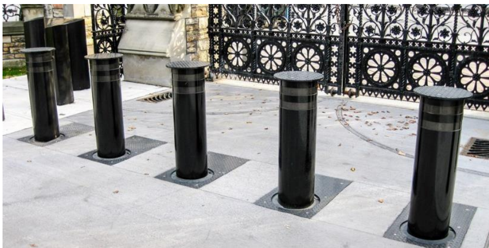
Fig. 2. Covering a larger opening with more retractable posts
