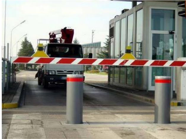
Fig. 1. Pillars to prevent the forced access to the barrier
