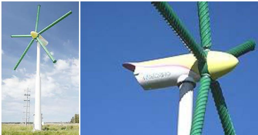
Fig. 6. Magnus wind turbine with fin-like on rotating cylinder blades [11]
