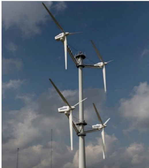
Fig. 3. Vestas multi-rotor wind turbine
