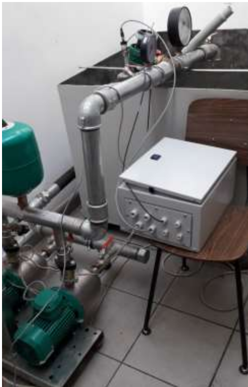
Fig. 6. Testing the injection device with differential piston under laboratory conditions
