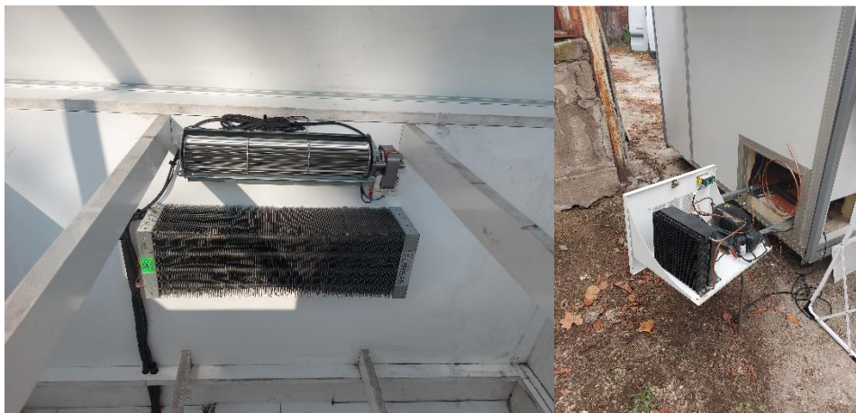
Fig. 9. Refrigeration installation subsystem
