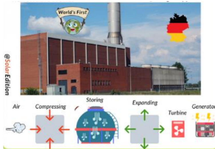
Fig. 1. Huntorf plant (Germany) and the principle of operation [2]
