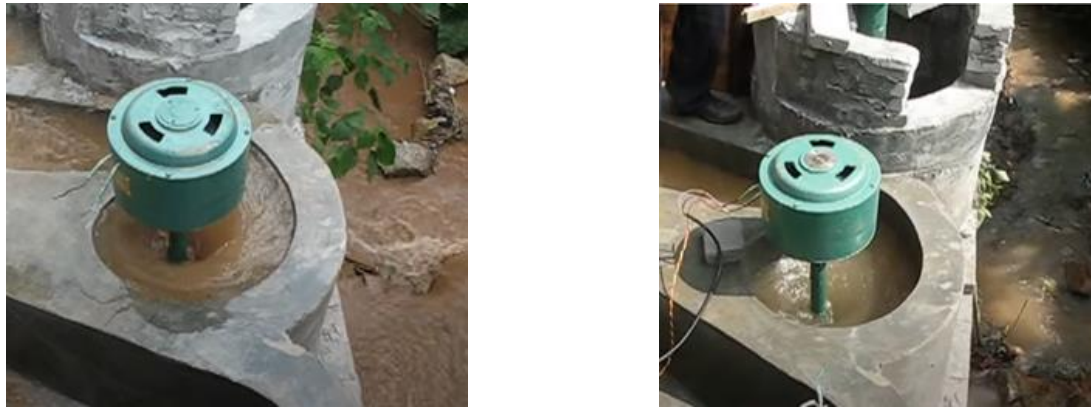
Fig. 2. Installation of low-head hydraulic turbines (at the head of the water drop)
