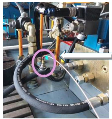
Fig. 4. Mounting accelerometers on the supply and return pipes (flexible pipes)
